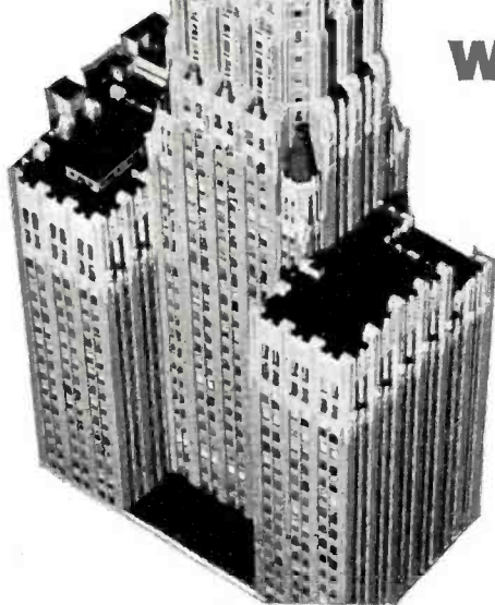
THE O'SULLIVAN BUILDING in the heart of downtown Baltimore, highest structure south of New York, offers WMAR a lofty perch for its FM Pylon and television Super Turnstile antennas.
